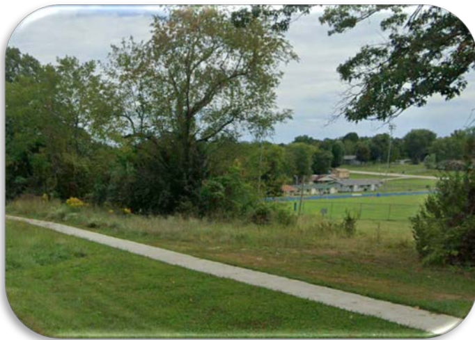
Sidewalk on south side of Rolla St./Hwy JJ.
