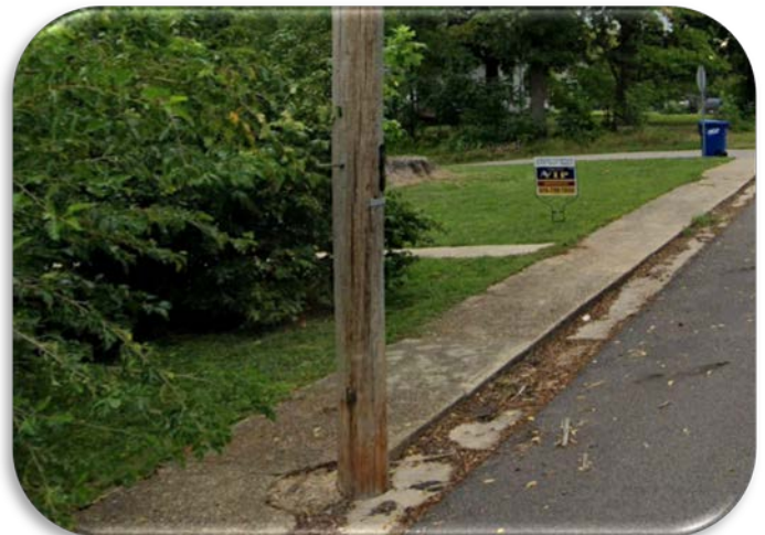
Sidewalk along north side of E. 10 th St.
